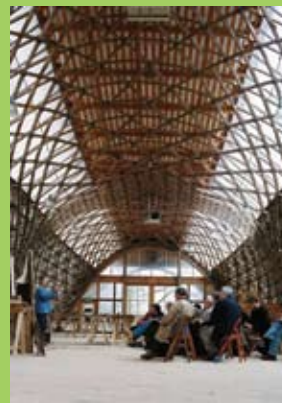
01 Downland Gridshell, built in 2002 for the Weald and Downland Open Air Museum. Edward Cullinan Architects
