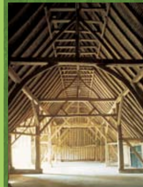
02 The Barley Barn, Essex c.1150-1200. Photograph: Will Pryce © Thames & Hudson, London, Ltd. from Architecture in Wood: A World History by Will Pryce, Thames & Hudson
